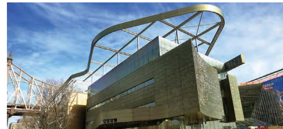
Northeast view of Cornell Tech’s Bloomberg Center, still under construction.
